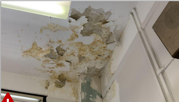
Failed plaster/interior finishes
