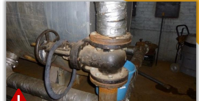
Failing heat distribution piping
