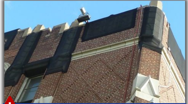
Temporary stabilization of brick erosion
