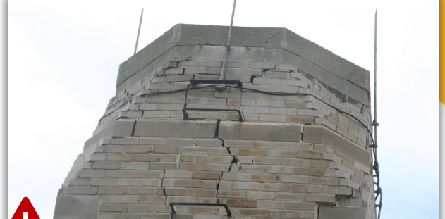
Displaced Chimney Masonry
